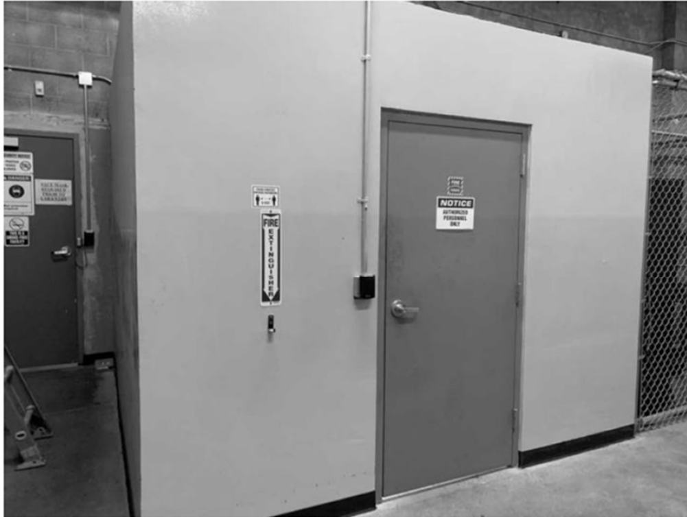
15 15-024 Date Taken: 8/12/2021 Vault room. Solid reinforced concrete with 2" solid steel door.
